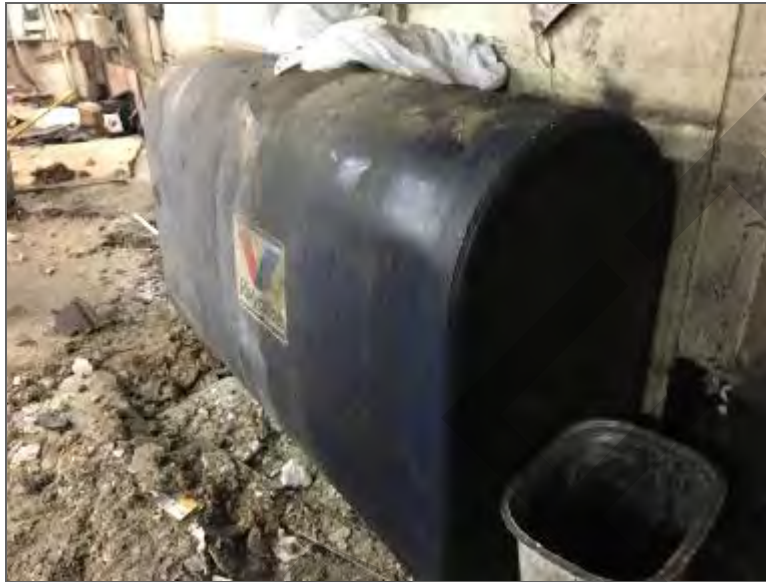
Photo 9 – A 910-L waste oil AST located along the south wall of the tenant space formerly occupied by Auto Re-Bex.
