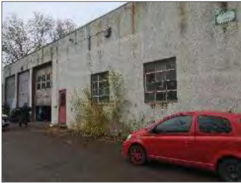
Asbestos-containing aggregate-embedded stucco present on the exterior walls of Garage 2 and Storage 2 at 320 McRae Avenue.
