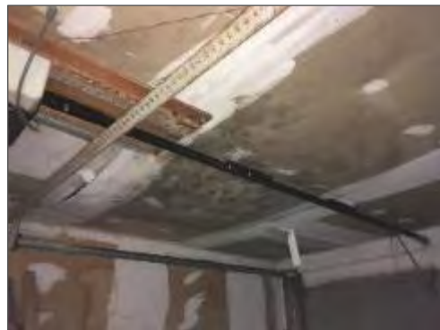
Mould present on the drywall ceiling in the separate Garage at 315 Tweedsmuir Avenue.
