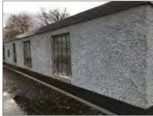
Asbestos-containing aggregate-embedded stucco present on the exterior walls of Storage 2 on the roof level at 320 McRae Avenue.
