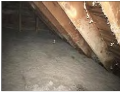
Non-asbestos spray-applied insulation present in the crawlspace (attic) at 311 Tweedsmuir Avenue.
