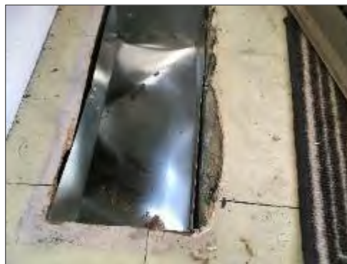
Asbestos-containing vinyl sheet flooring present as the base layer in the front entrance at 311 Tweedsmuir Avenue.
