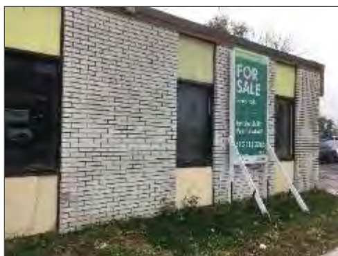
Asbestos-containing cement board present above and below the windows along Office 1 & 2 at 320 McRae Avenue.
