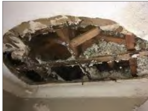
Mould present on the back side of the drywall/textured plaster ceiling finish in the front entrance at 315 Tweedsmuir Avenue.
