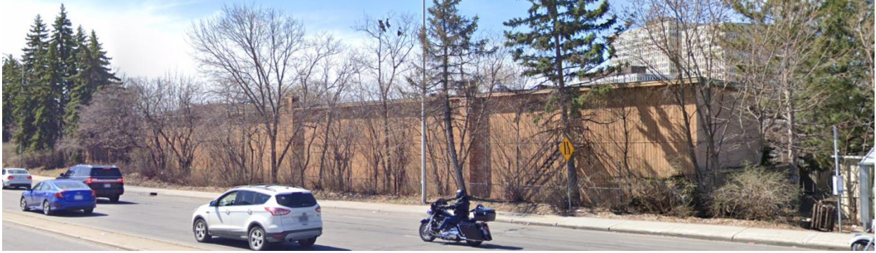
View looking south-west along the Vanier Parkway showing the back side of the now demolished motel. The Esso Station is located at the far right edge of the image.
