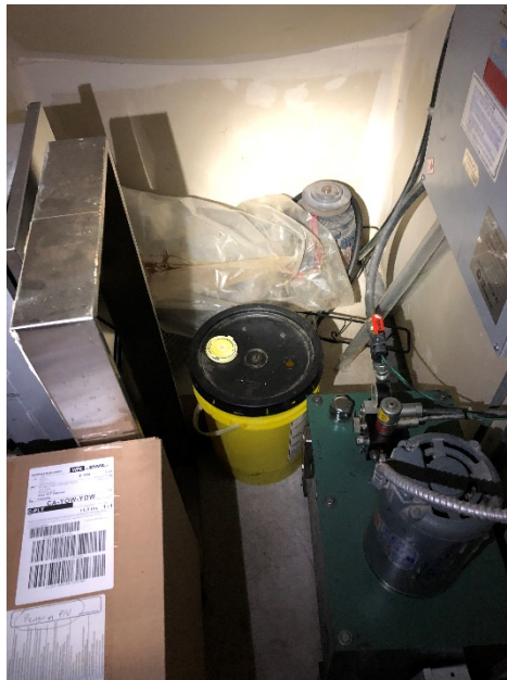
4. Photograph of the hydraulic elevator pump (bottom right) and pail of hydraulic oil (1/4 full)
