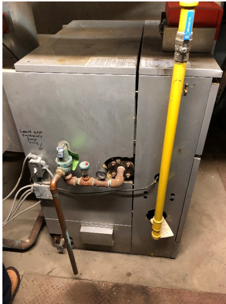
5. Natural gas boiler, located in basement of the church
