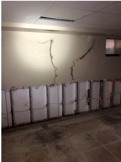
9. Basement of 9 Parkmount Crescent; visible signs of mould can be seen on some walls.
