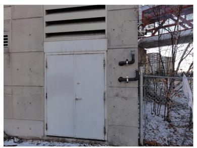
Photo 14- View of vent and fill pipes associated with back-up power generator located adjacent southeast of the Site, associated with OC-Transpo station .
