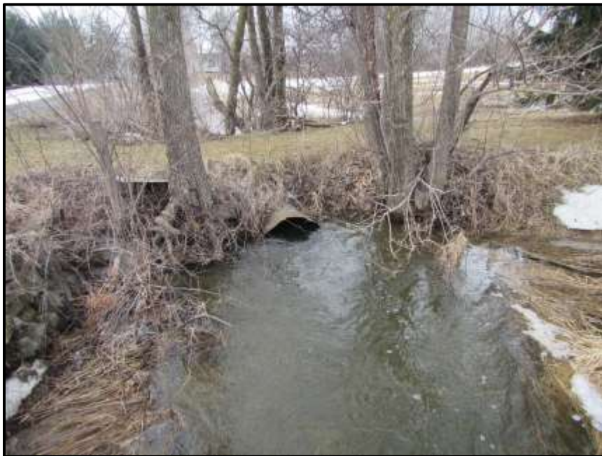
Photograph 4: Survey Site #1 - 60 cm CSP culvert under the driveway west of March Road (facing upstream) (March 30 th , 2018).
