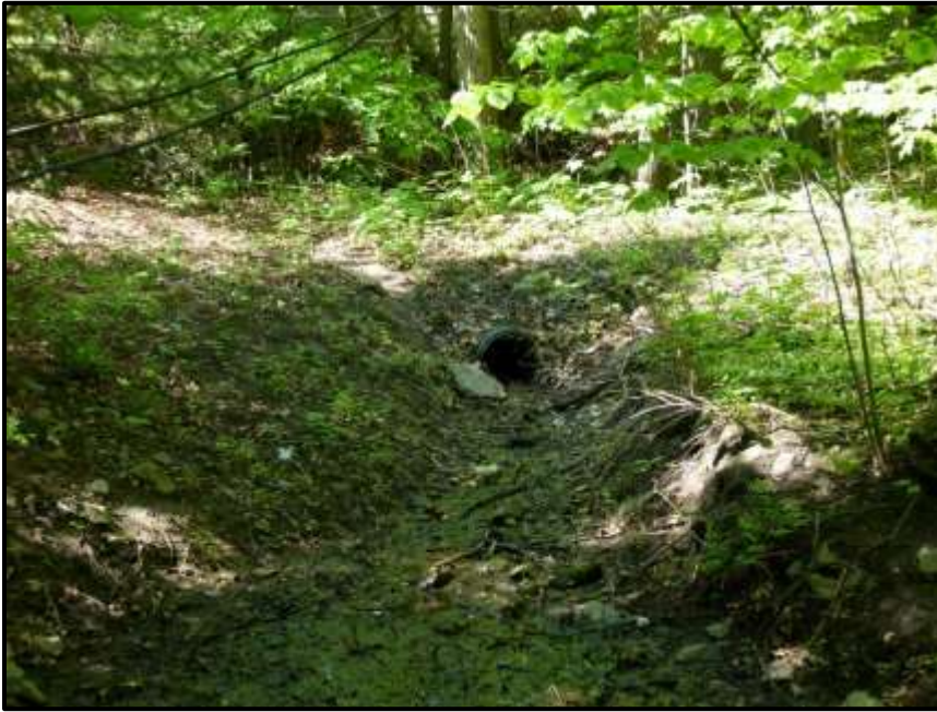
Photograph 111: Pipe from the adjacent subdivision that feeds water into the Stormwater Infiltration Swale within Section #6 (May 24 th , 2018).
