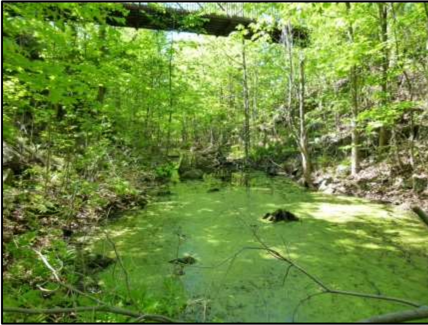
Photograph 110: Stormwater Infiltration Swale within Section #6. The Stormwater Infiltration Swale is fed by a pipe from the adjacent subdivision. The Section #6 Stormwater Infiltration Swale has no outlet, and standing water infiltrates/evaporates (May 24 th , 2018).
