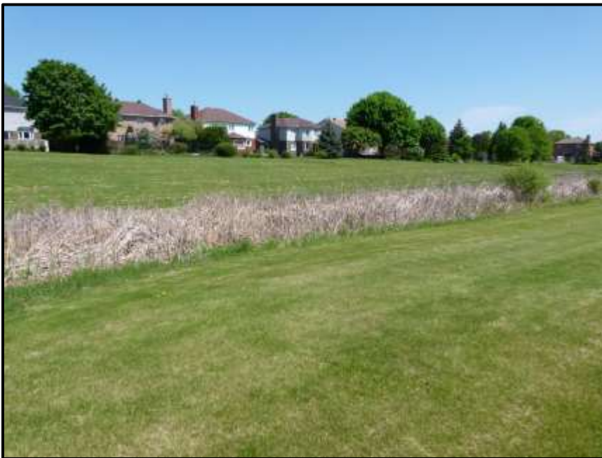
Photograph 112: Dry Stormwater Infiltration Swale within Section #3 – no surface water observed (May 24 th , 2018).
