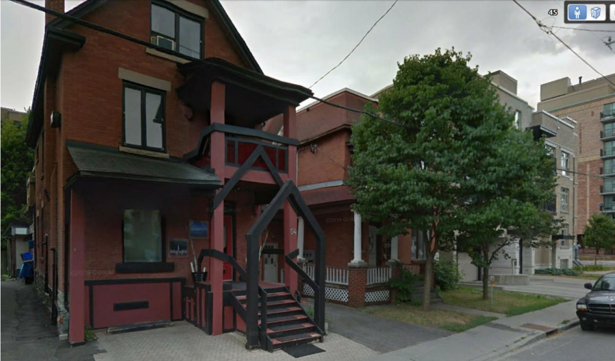
Figure 4: View of the development site 58 Florence to the right concealed behind the trees, and 54 Florence to the left.
