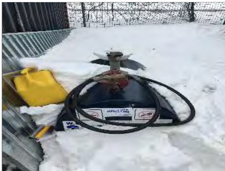
Photo 6 – Diesel AST located exterior to the west elevation of the Site Building (PCA).
