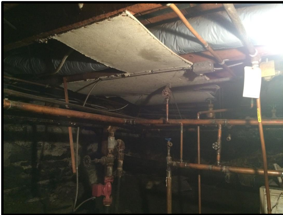
Photograph 4: View of suspected asbestos containing insulation board fastened to floor joists within the basement of 72-74 St. Andrew Street.
