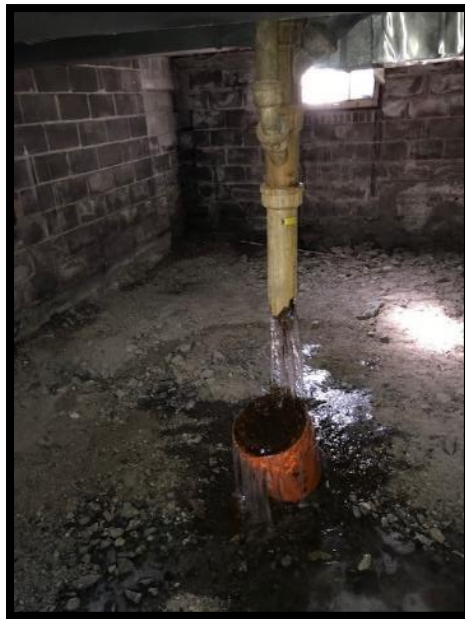
Photograph 10: View of broken water pipe in the southeast corner of the basement of the Site building (March 2019).
