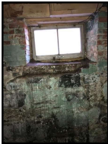
Photograph 12: View of the southwest basement window with water trickling into basement (March 2019).
