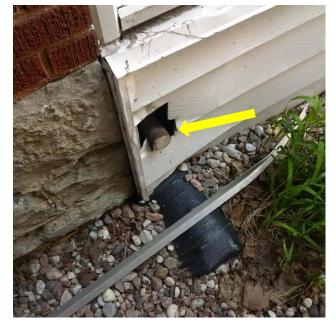
Photograph No. 5 View of previous AST fill pipe at northwestern corner of site building
