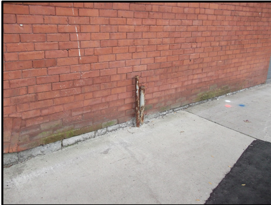
Photograph 7: Photo illustrates vent and fill pipes along the north wall of the commercial building (fronting onto Frank Street) adjacent to the west of the Phase I Property, facing southwest.
