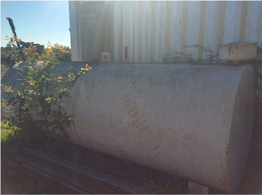
Photo 11: View of an actively used AST (APEC 2B) on the Equipment Storage Area occupied by M-Roc Ltd. No staining/odour observed. Facing northeast.
