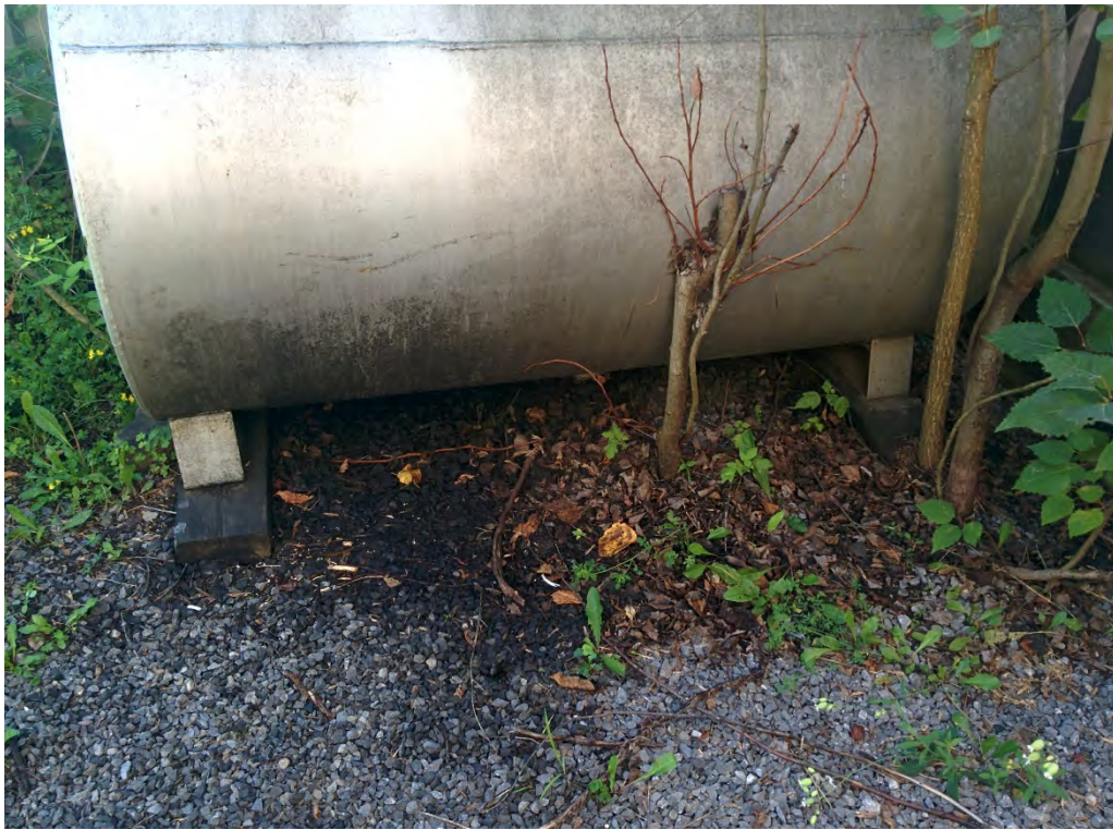
Photo 13: View of an actively used AST (APEC 2C) on the Equipment Storage Area occupied by M-Roc Ltd. Slight staining and odour observed. Facing northeast.
