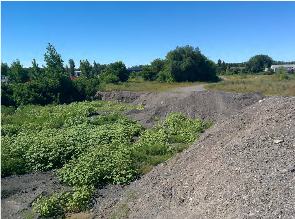
Photo 16: View of imported fill area immediately northeast of the Equipment Storage Area. The area consists of coarse granular material. Facing southeast.
