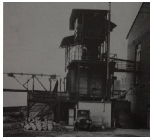
15. Two-ton byproduct coke oven, Fuel Research Laboratories, 1931 (Source: Ignatieff, 1981).
