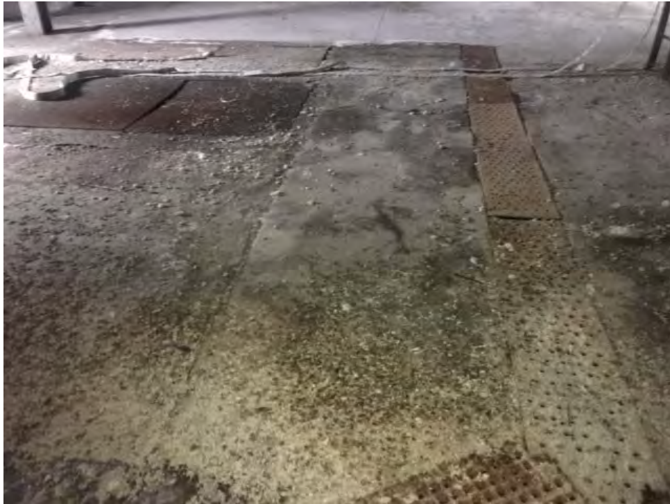
Photo 25: Potentially asbestos-containing fibres observed on the floors of the building at 552 Booth Street.
