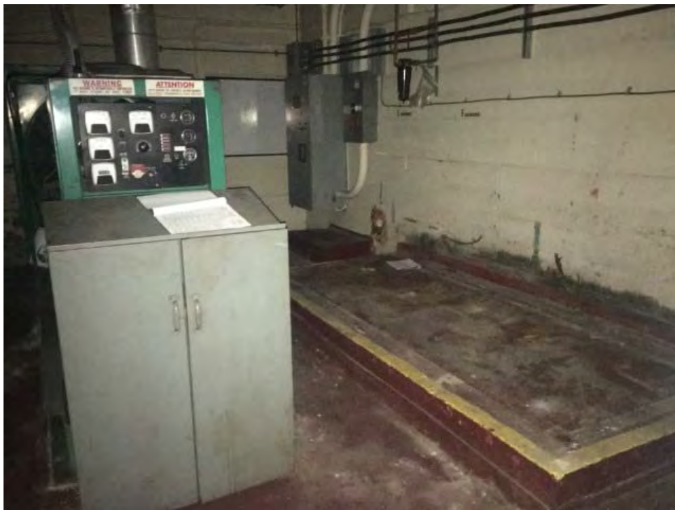
Photo 2: Photo of the generator and likely location of former day tank in the northeast corner of the central heating plant.
