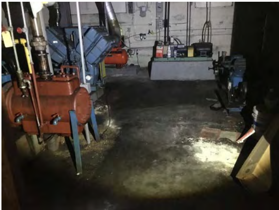
Photo 34: Oil absorbent located beneath a compressor adjacent to a floor drain in the southeast corner of the basement of the 550 Booth Street building. Other mechanical equipment is visible in this room.
