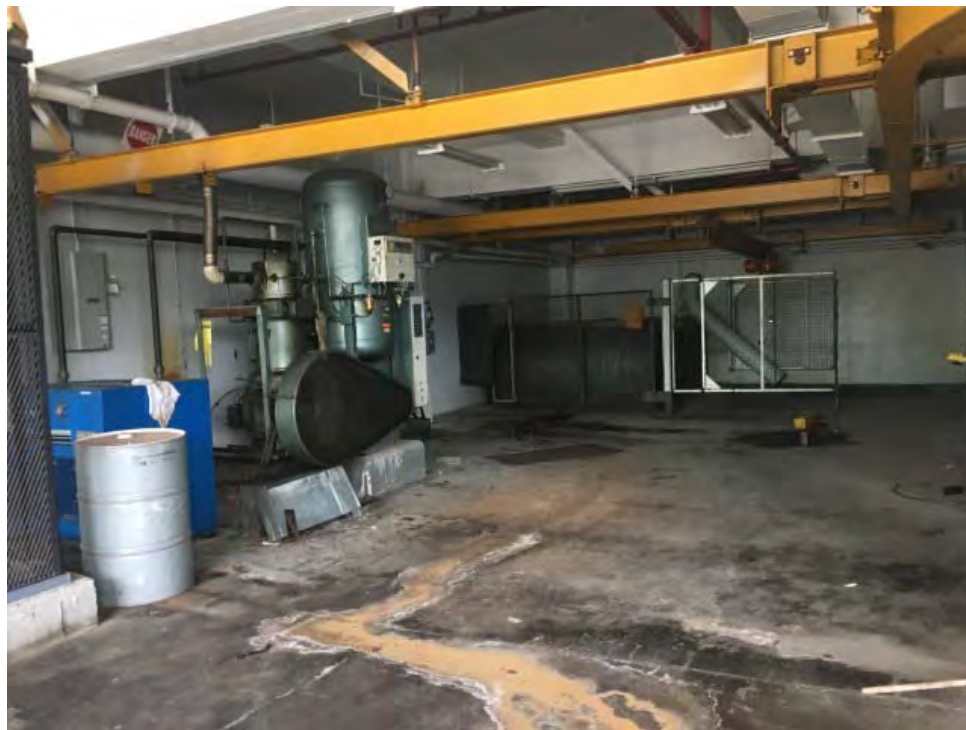
Photo 44: Compressor, air dryer and drum of ethylene glycol in the sub-basement of 556 Booth Street. Absorbent and staining was observed near the compressor.
