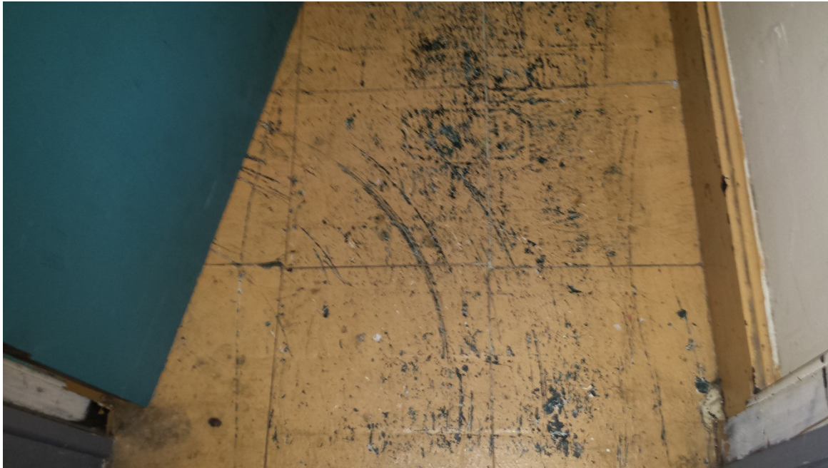
Photograph 5: Vinyl floor tile in poor condition at 423/425 McLeod Street.
