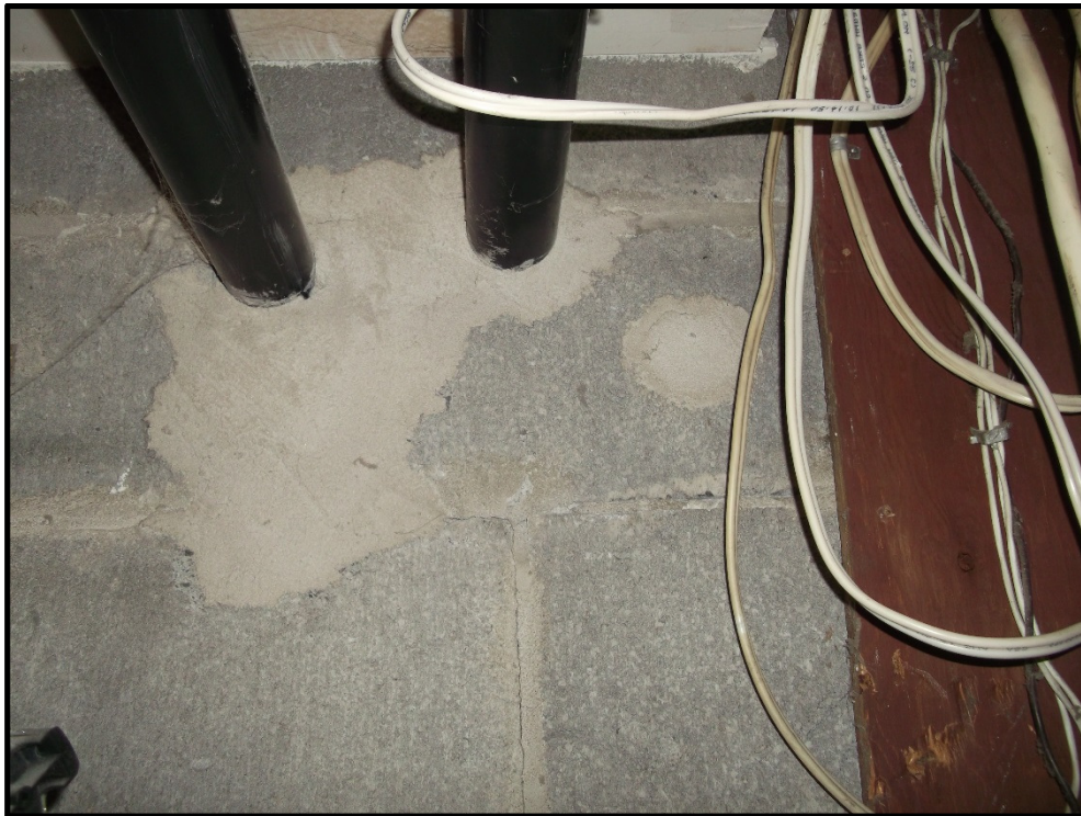
Photograph 10: Possible location of former vent and fill pipes leading to interior AST at 974 Fisher Avenue.
