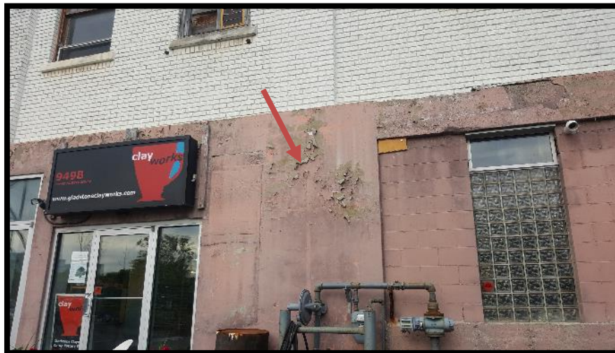
Photograph 8 – View of peeling paint (see arrow) on the exterior of the Site building associated with 951 Gladstone Avenue.
