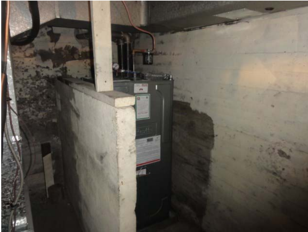
Photo 19: View of the double walled AST for furnace oil storage located in the basement of 431 Ravenhill Avenue (photo taken Sep. 11, 2018).
