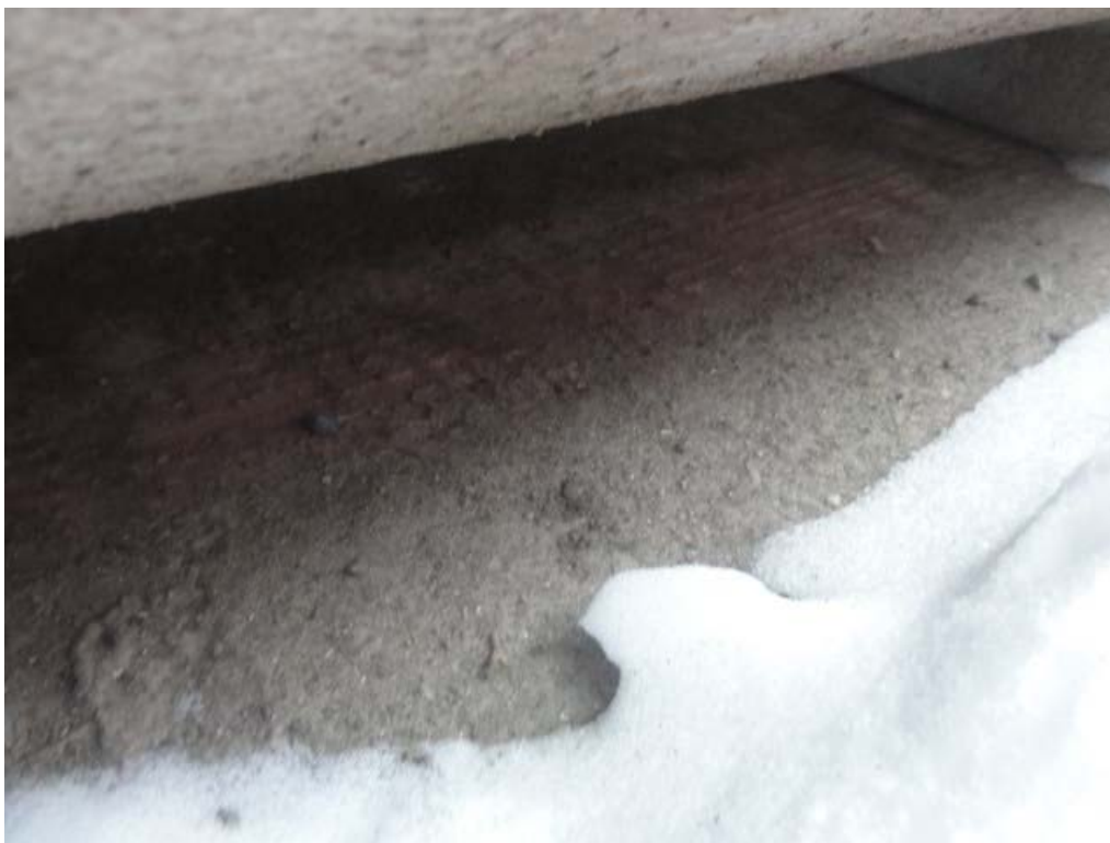
Photo 10: View of the visible portion of the concrete pad underneath AST showing no evidence of stain/spills (photo taken Jan 4, 2018).
