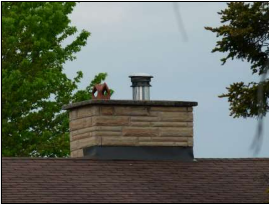
Photograph 31: Chimney at 1015 March Road. Note metal cap and ceramic liner (May 24 th , 2017).
