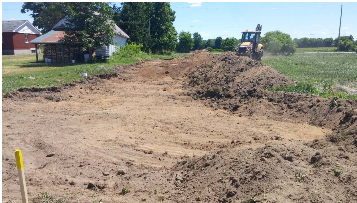
Image 8: Backfilling in eastern half facing southeast.
