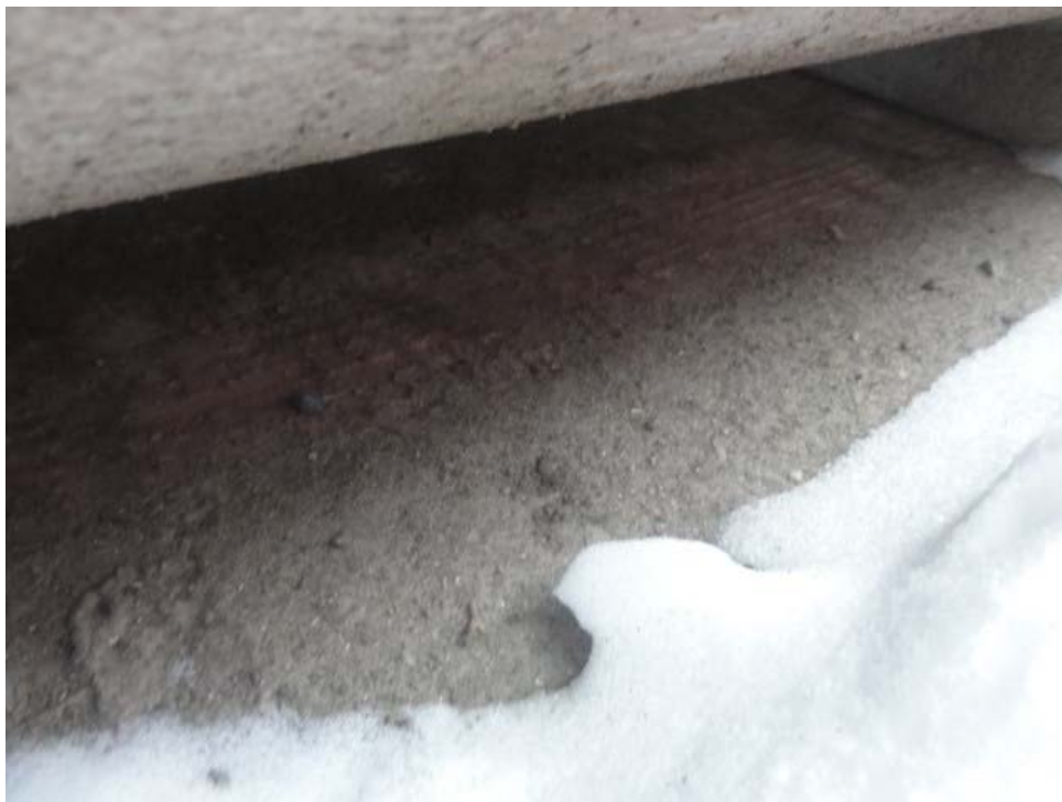
Photo 10: View of the visible portion of the concrete pad underneath AST showing no evidence of stain/spills.
