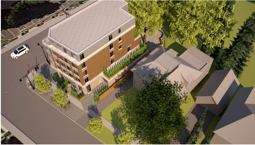
Figure 23: A one storey attached accessory building is set back 5.2 m from Clemow Avenue and at its narrowest point .9 m from the property line. Accessed from double doors, the building will provide bicycle parking and garbage/recycling storage. The roof will be treated as a green roof with plantings.
