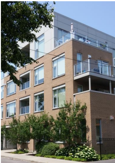
Figure 11: 621-625 Bank Street at the corner of Patterson Avenue looking north. The four-storey building is a comparable mixed-use building with the double height fourth floor taking the building to the 15 m allowable height. The stepped east elevation next to the existing residential creates a comfortable transition to the next-door neighbor. Credit: Commonwealth.
