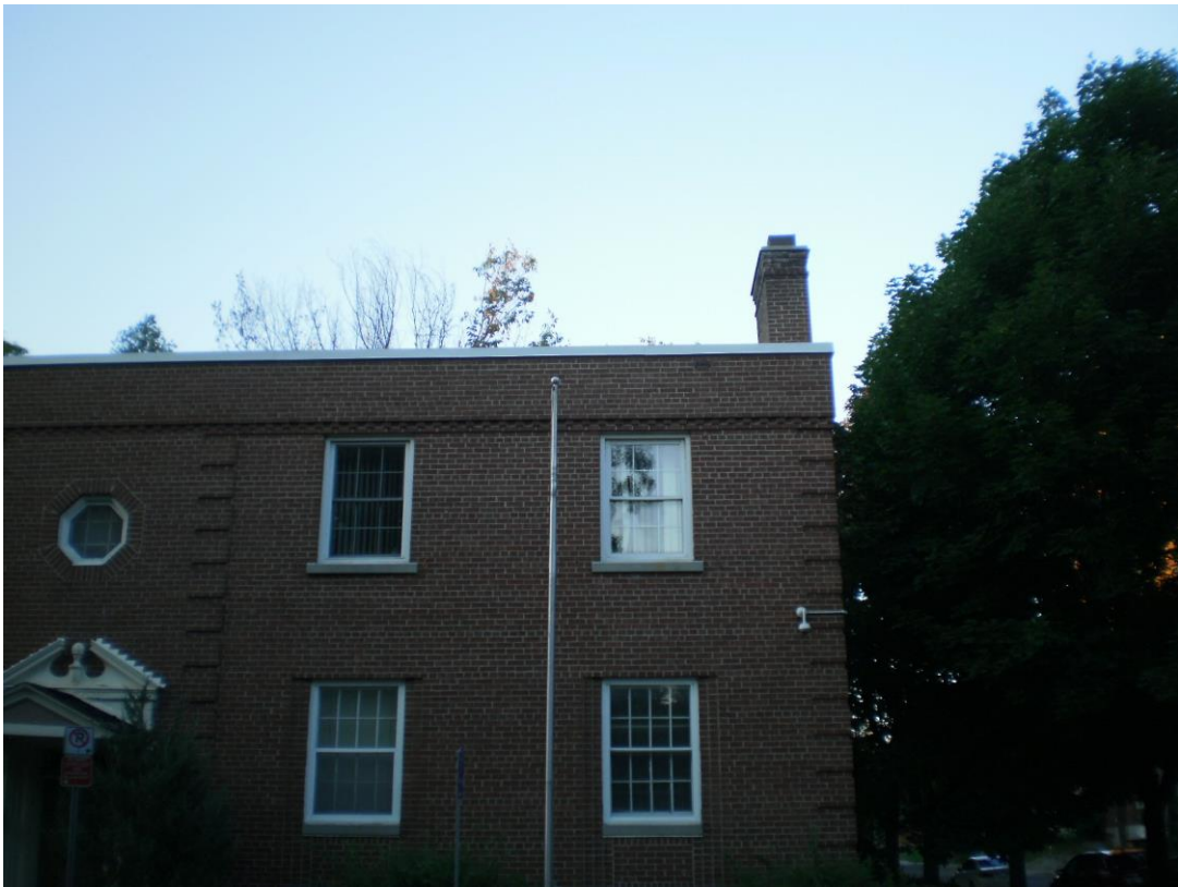
Photo 2 – South half of the building at 231 Cobourg Street with the chimney on south face of the building
