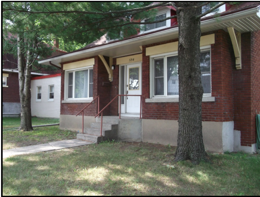
Photograph 9: View of east face of 534 Edison Avenue and the addition adjoining to 540 Edison Avenue, facing southwest.
