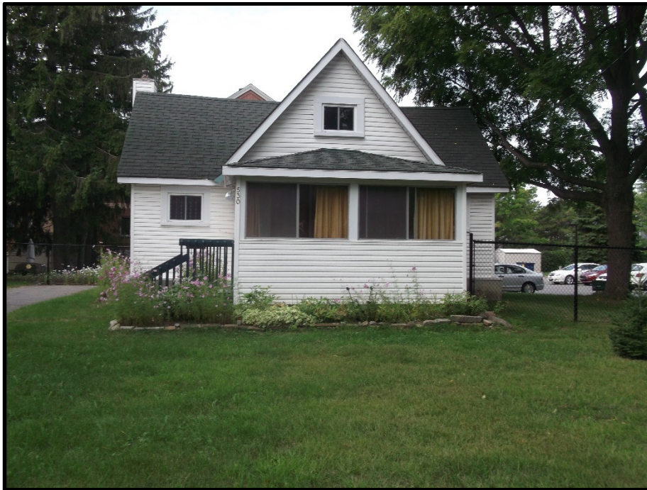
Photograph 8: View of the east face of 530 Edison Avenue, facing west.
