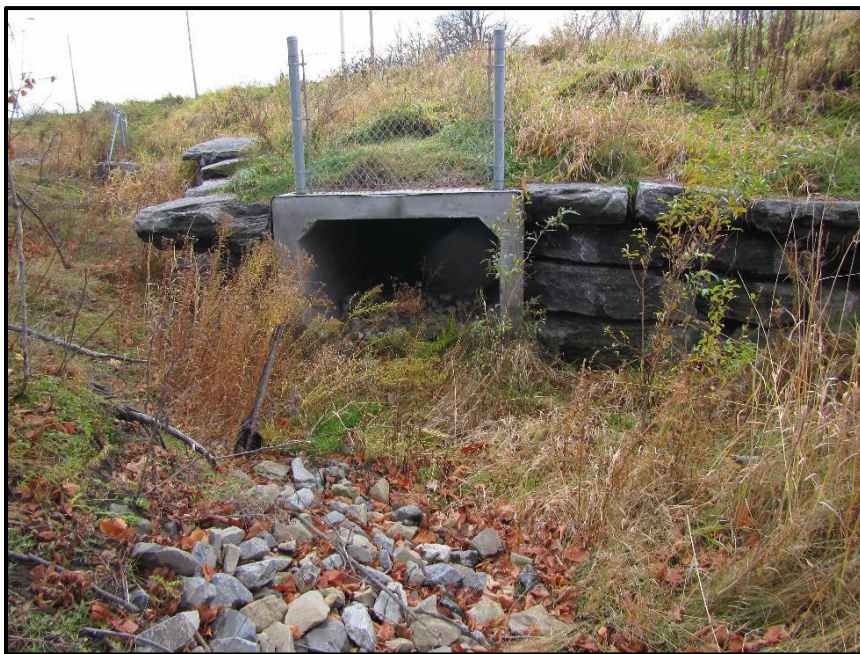
Photograph 26: Culvert at Terry Fox Drive, looking west (November 16 th , 2016).
