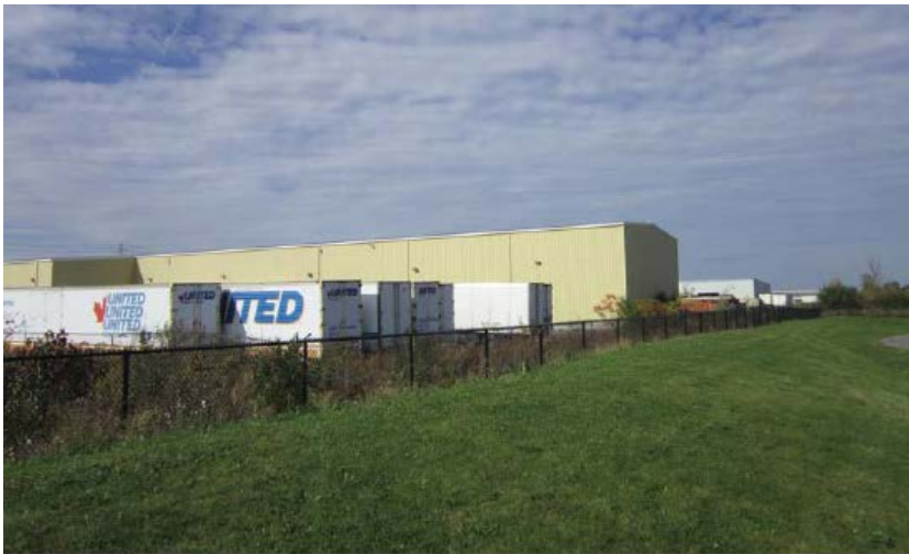
Photo 3: Industrial uses to the west of the site.
