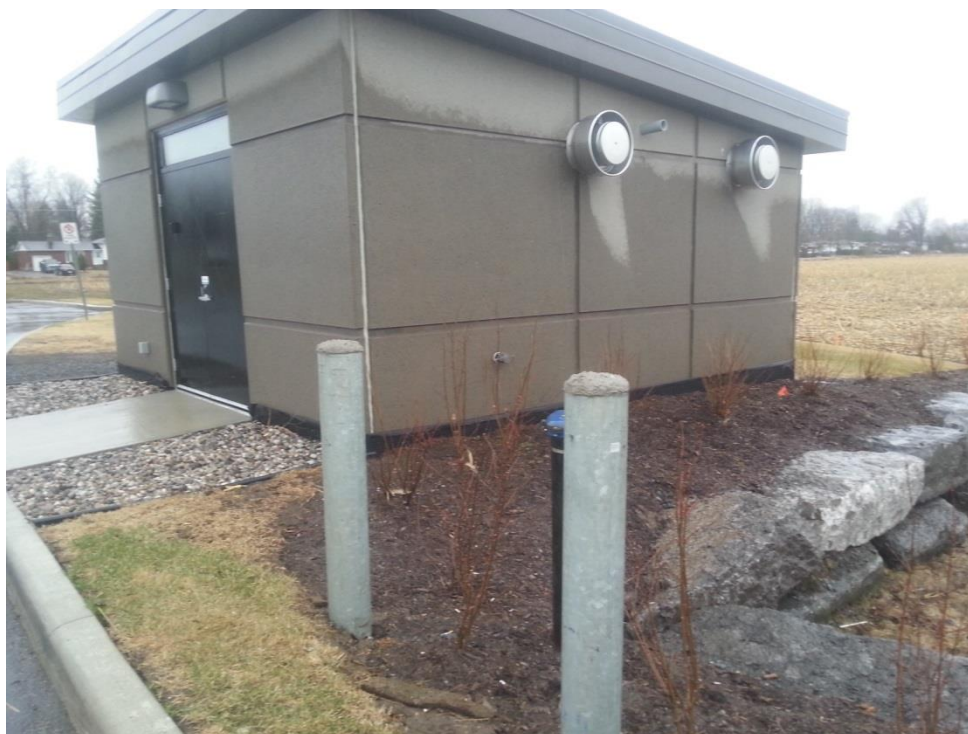
Photograph 10: Off-Site utility building at the grocery store property.
