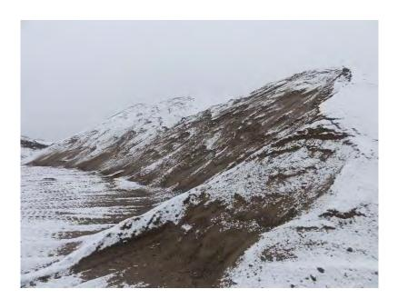
Photo 14 – Excavated materials stockpiled (following screening) as clean sand on the eastern portion of the Site.
