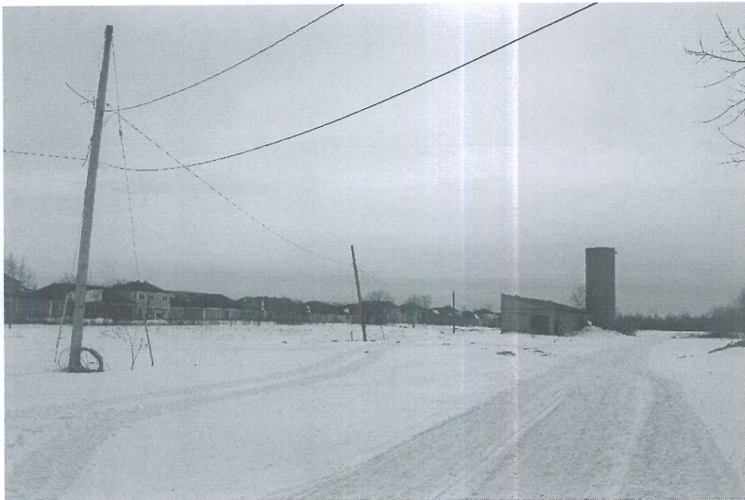
Storage Building and Silo
