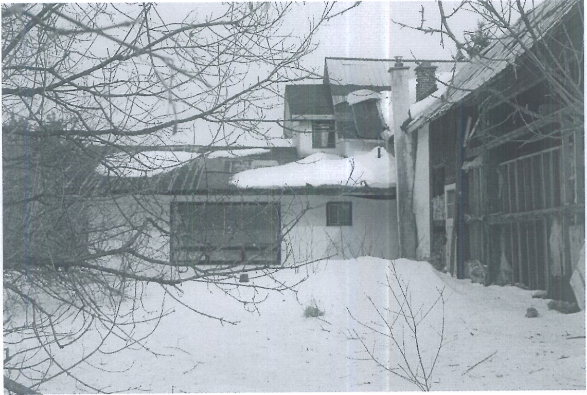
South Side of Barn Building
