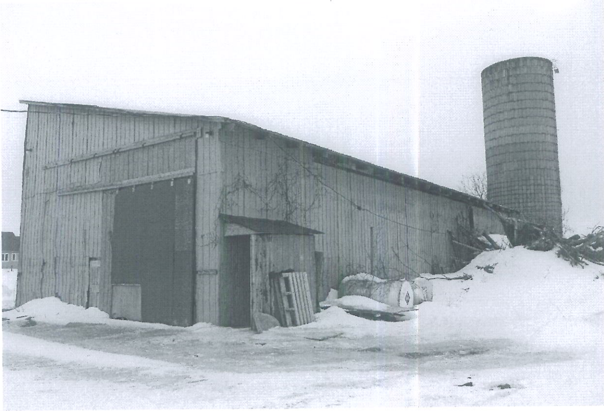
North Side of Existing Storage Building and Silo
