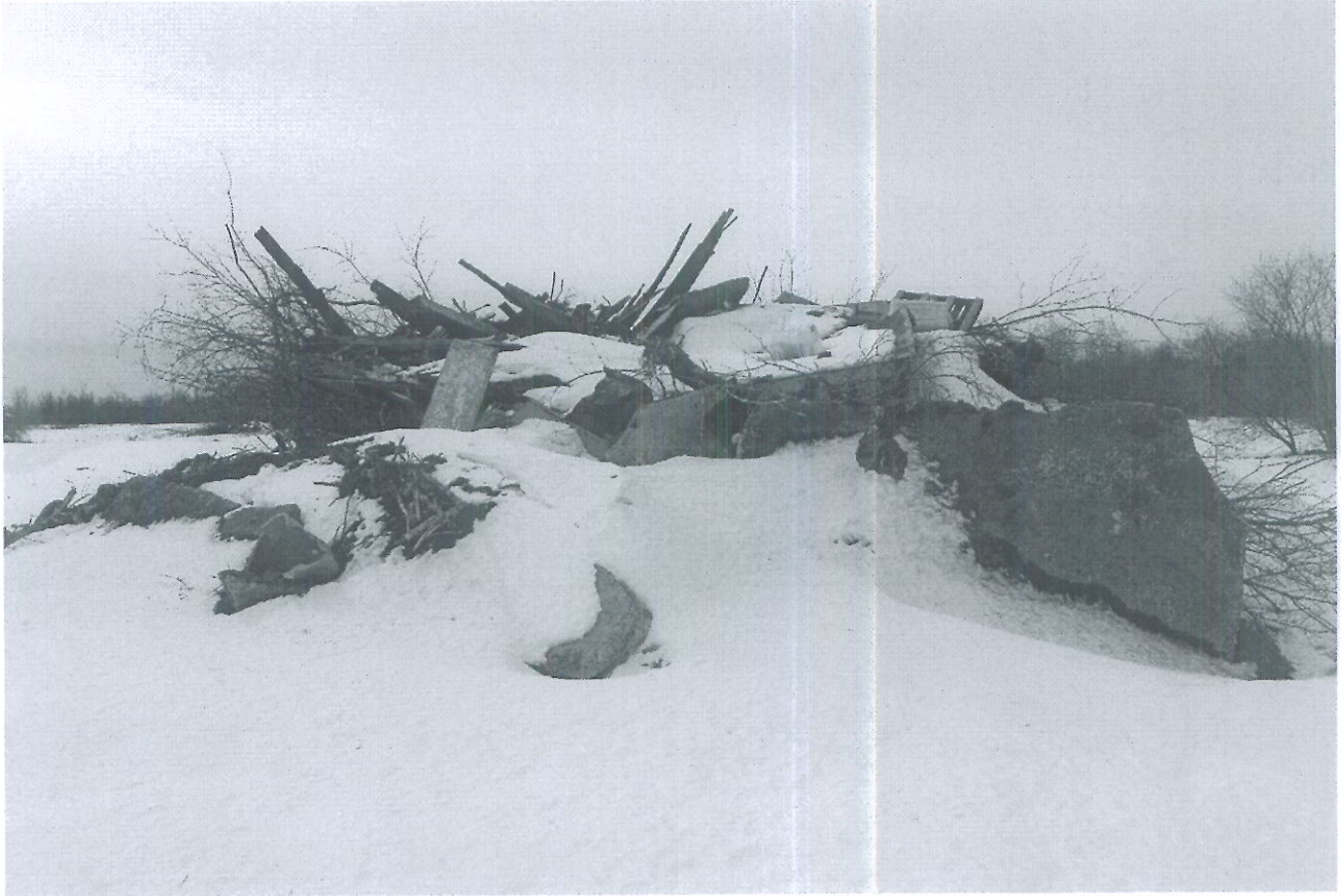
Miscellaneous Fill Debris in East Portion of Site
