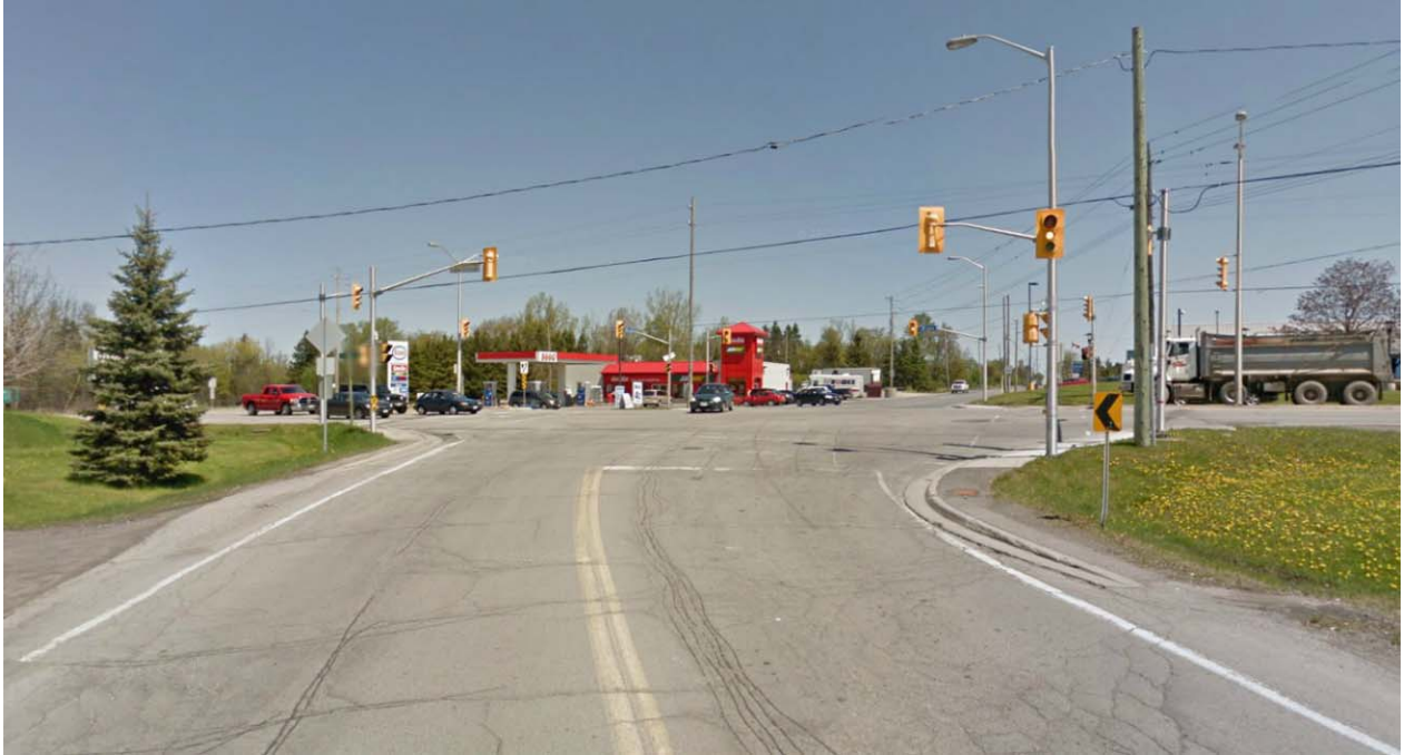
Bank & Leitrim – Eastbound on Leitrim Road
