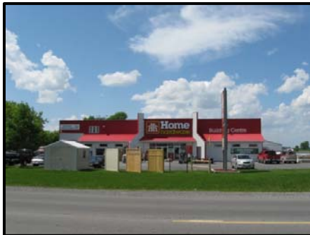
Home Hardware (just west of the northern parcel)
