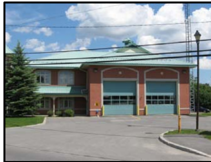
Local Fire Hall (just east of the southern parcel)
