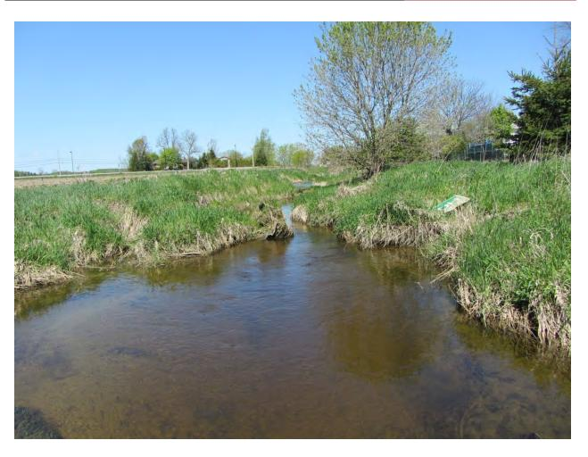
Section 2 is also located in Reach 3 and is located upstream of the Fortune Street culvert where the Drain takes an abrupt, 90-degree turn. The outside bank is rapidly eroding at this site and the section is, as seen in the section plot below, trying to adapt to the high sediment inputs.
