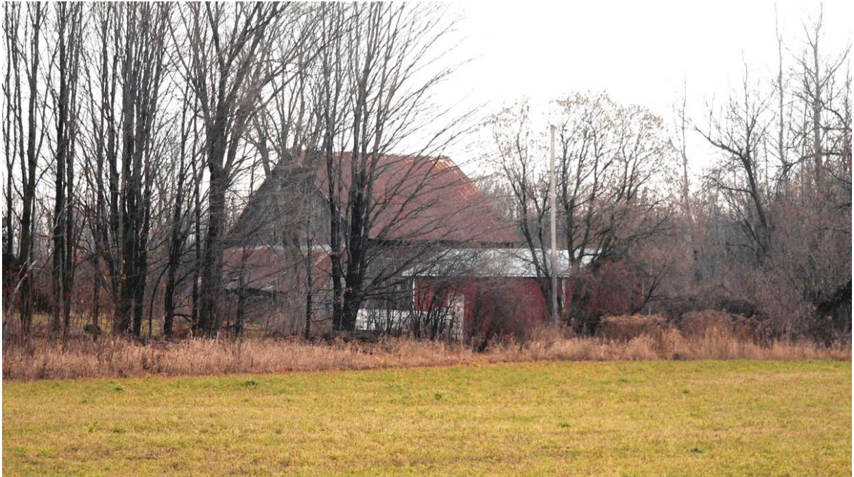
Plate 5: Barn and outbuildings to the rear of the current dwelling at 1730 Wilhaven Drive.
