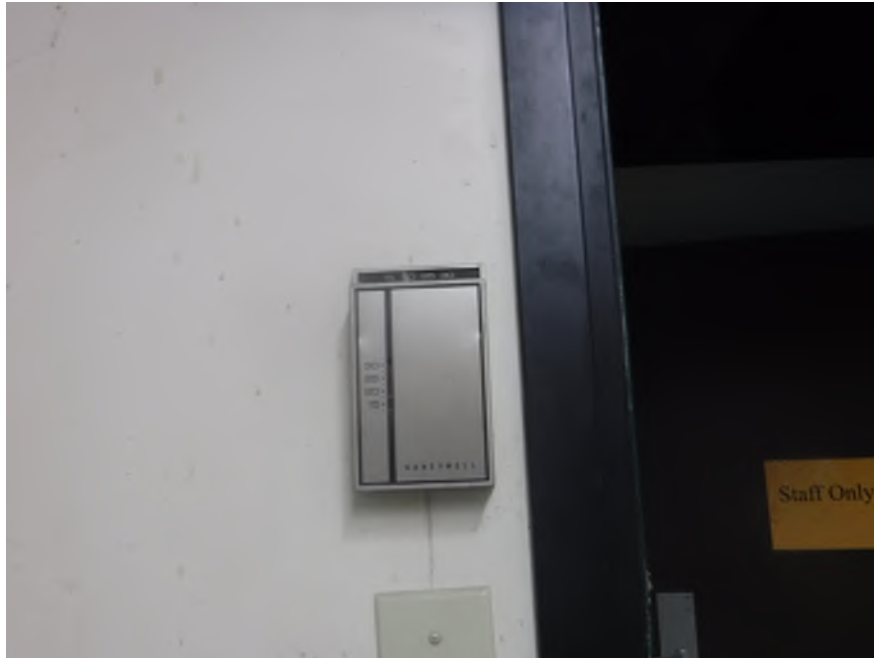
Photo 23. Representative photograph of suspect mercury-containing thermostats located throughout the building #5.
