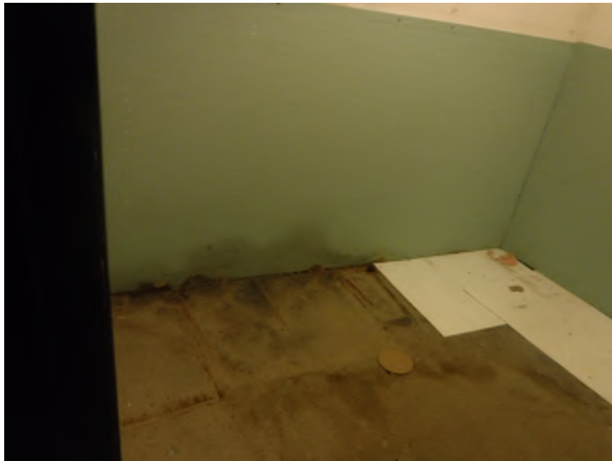
Photo 26. Suspect mould and water damage located in a room located in the northeast corner of building #5.
