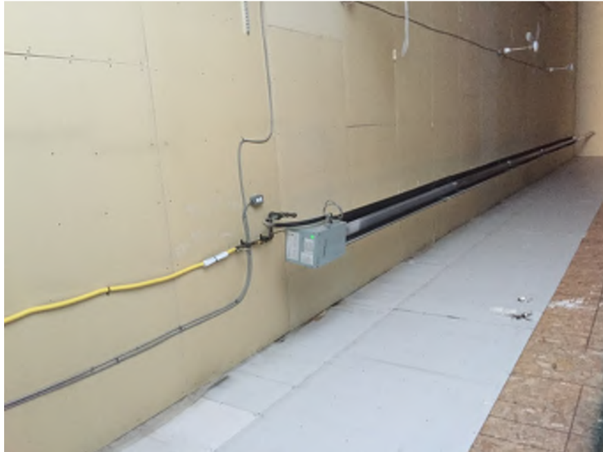
Photo 32. Natural gas heater located on the south side of shed #2.
