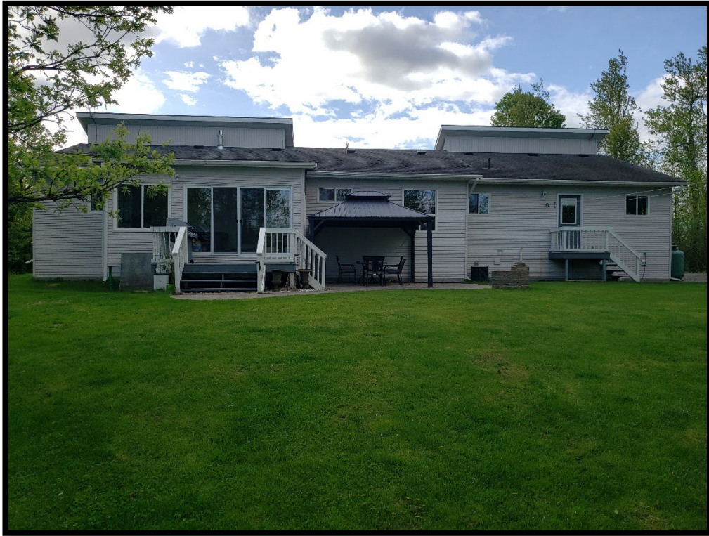
Figure 1: General view of back of house within study area (MH1511-D015).
