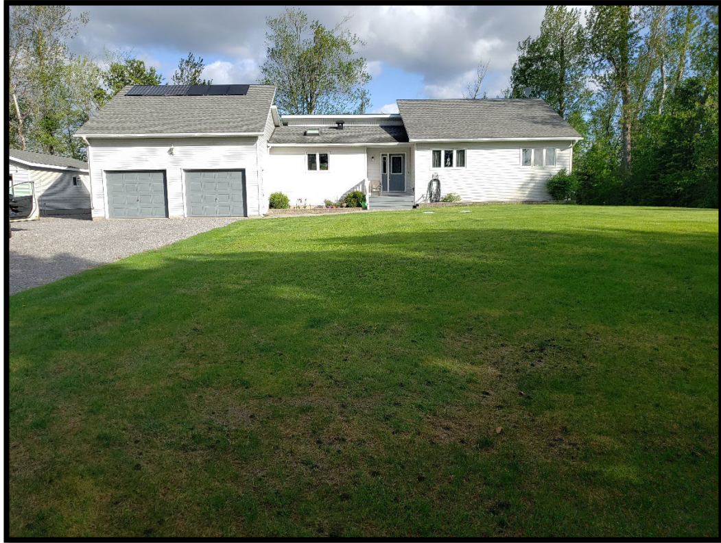
Figure 9: View of the front of the house showing the raised land of the septic bed (MH1511-D002).
