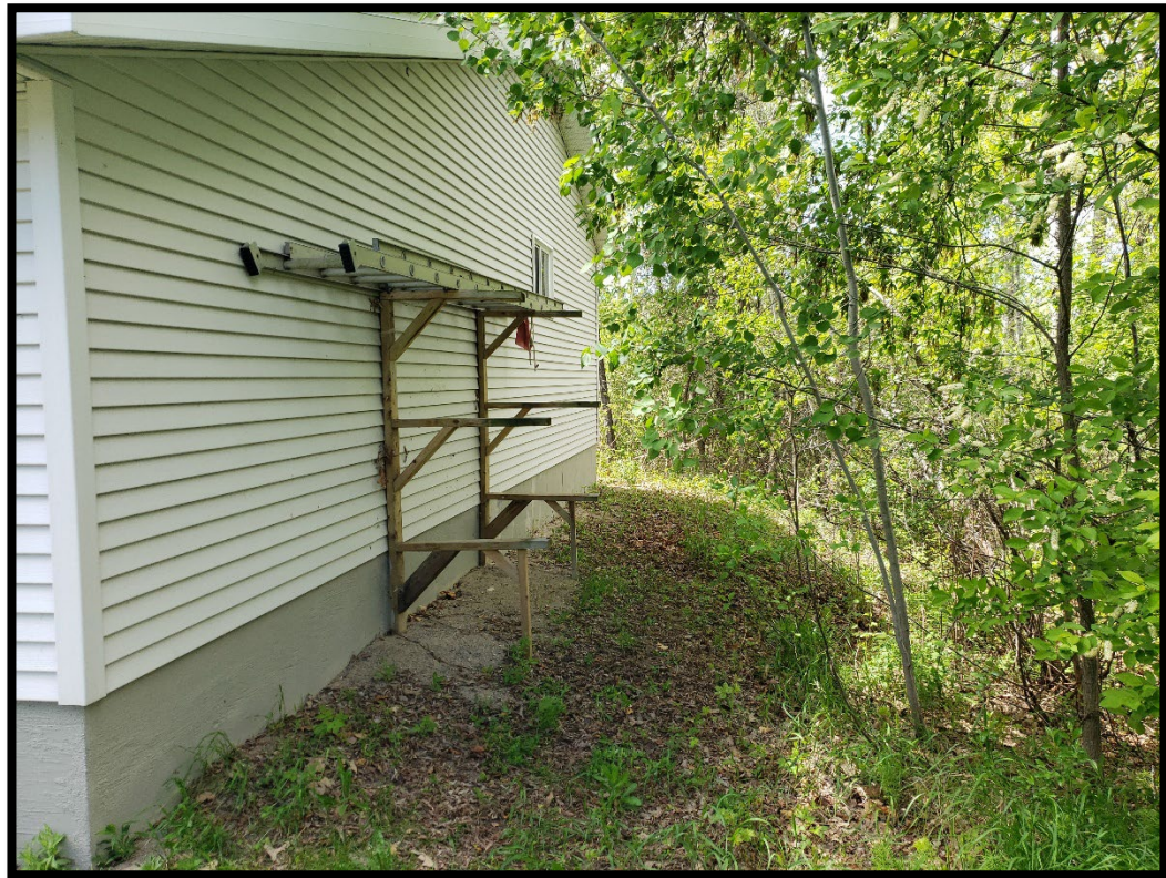
Figure 8: Example of structure with landscape built up around it (MH1511-D037).
