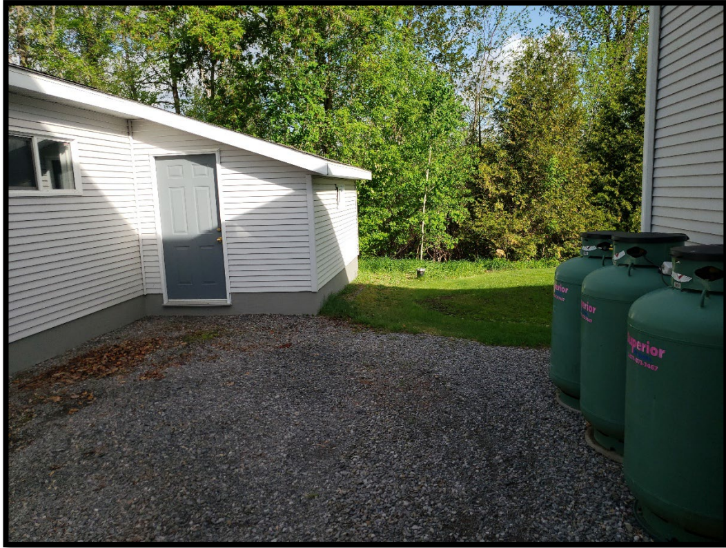
Figure 7: Example of structures and utilities on the property (MH1511-D012).
