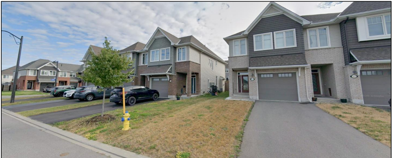
Figure 4: Abutting the Subject Site to the east is a low-rise, residential subdivision (Google Streetview, 2025).
