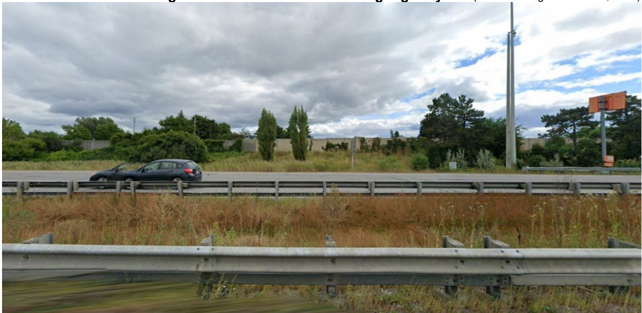
Figure 4: South of the site showing Highway 174 (Source: Google Streetview, 2025)
