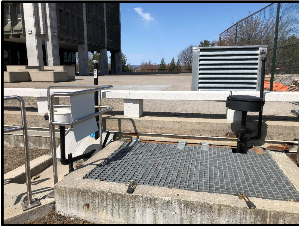
Photograph 3: View of the vent and fill pipes on the south face of the Brooke Claxton building, facing north.
