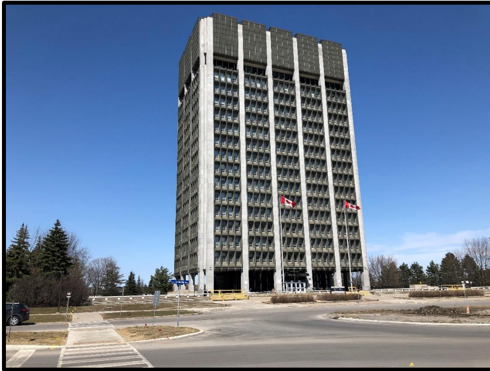
Photograph 1: View of the front of the Brooke Claxton building, facing north.
