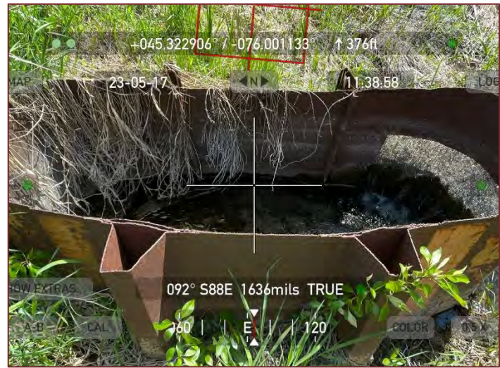
Site Photograph 6: The vertical drain on-site.
