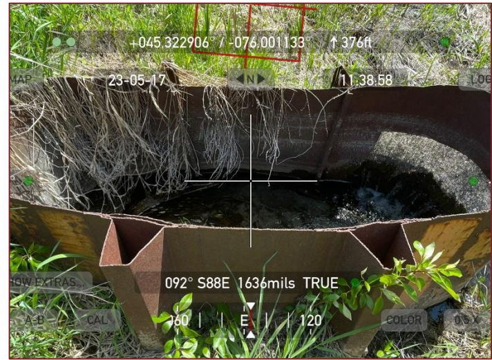
Site Photograph 6: The vertical drain on-site.
