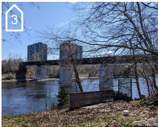
Figure 6: View 3 on key map looking southeast from the eastern edge of the site.
