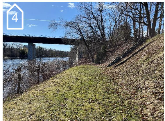
Figure 7: View 4 on key map looking south of the eastern edge of the site.
