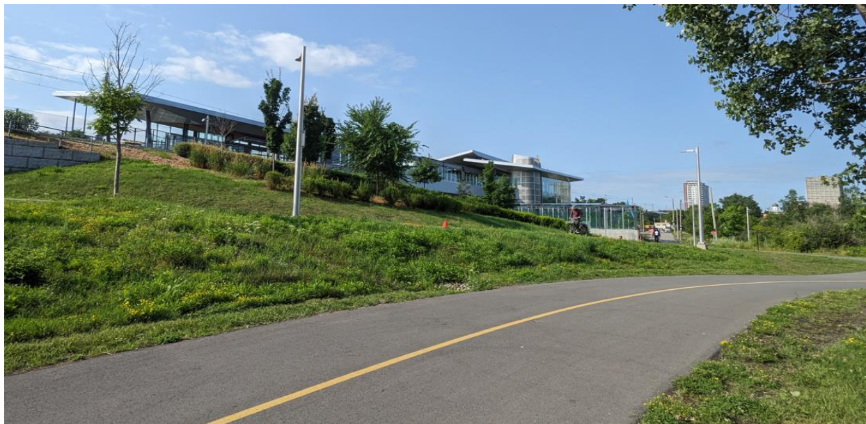
Figure 5. Bayview Station looking southwest from the multi-use pathway within LeBreton Flats.
