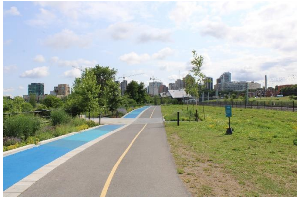
Photo 4.11: Multi-use pathway looking east towards Pimisi Station
