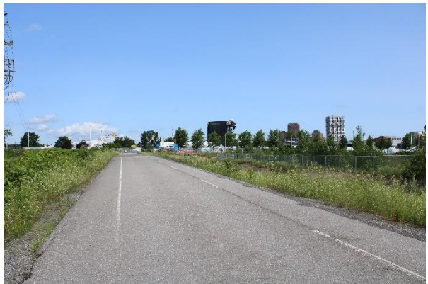
Photo 4.9: Unexcavated Vimy Place roadway north of Wellington Street
