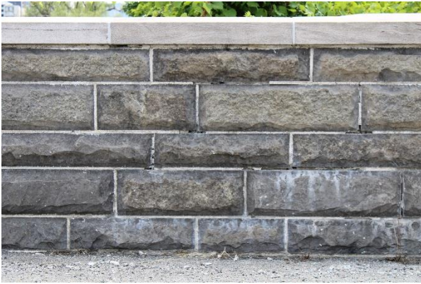
Photo 4.23: Broad Street Bridge stone detail
