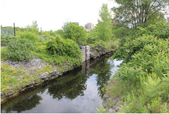
Photo 4.17: Open Aqueduct looking east
