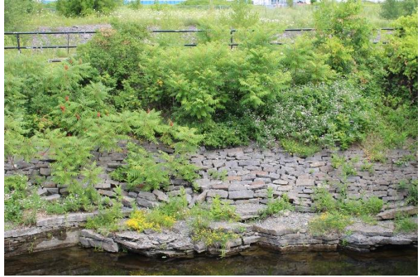
Photo 4.18: North wall of Open Aqueduct
