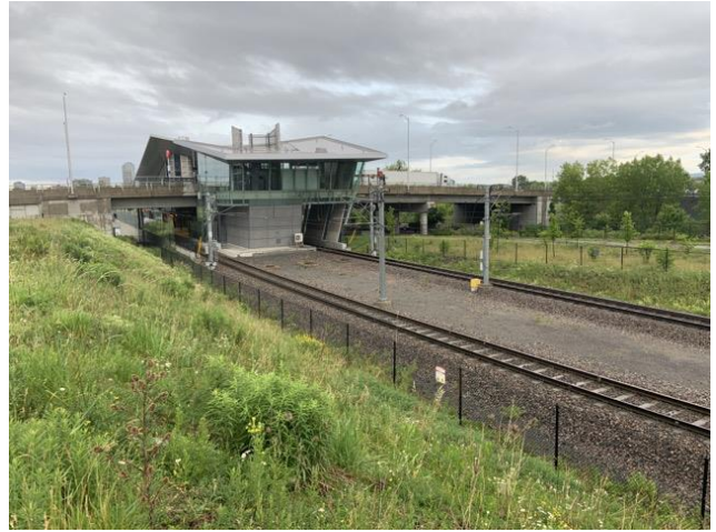
Photo 2: LRT east of Pimisi station and Booth Street in CVI_1, facing northwest.
