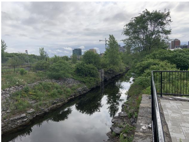
Photo 11: Fleet Street Tailrace in OA (Open Water), facing east.
