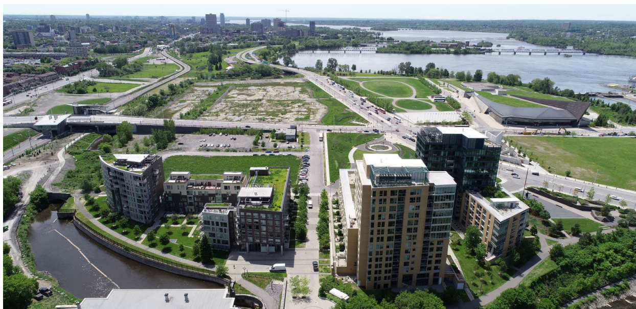
Figure 1-1: Aerial View of LeBreton Flats 2
