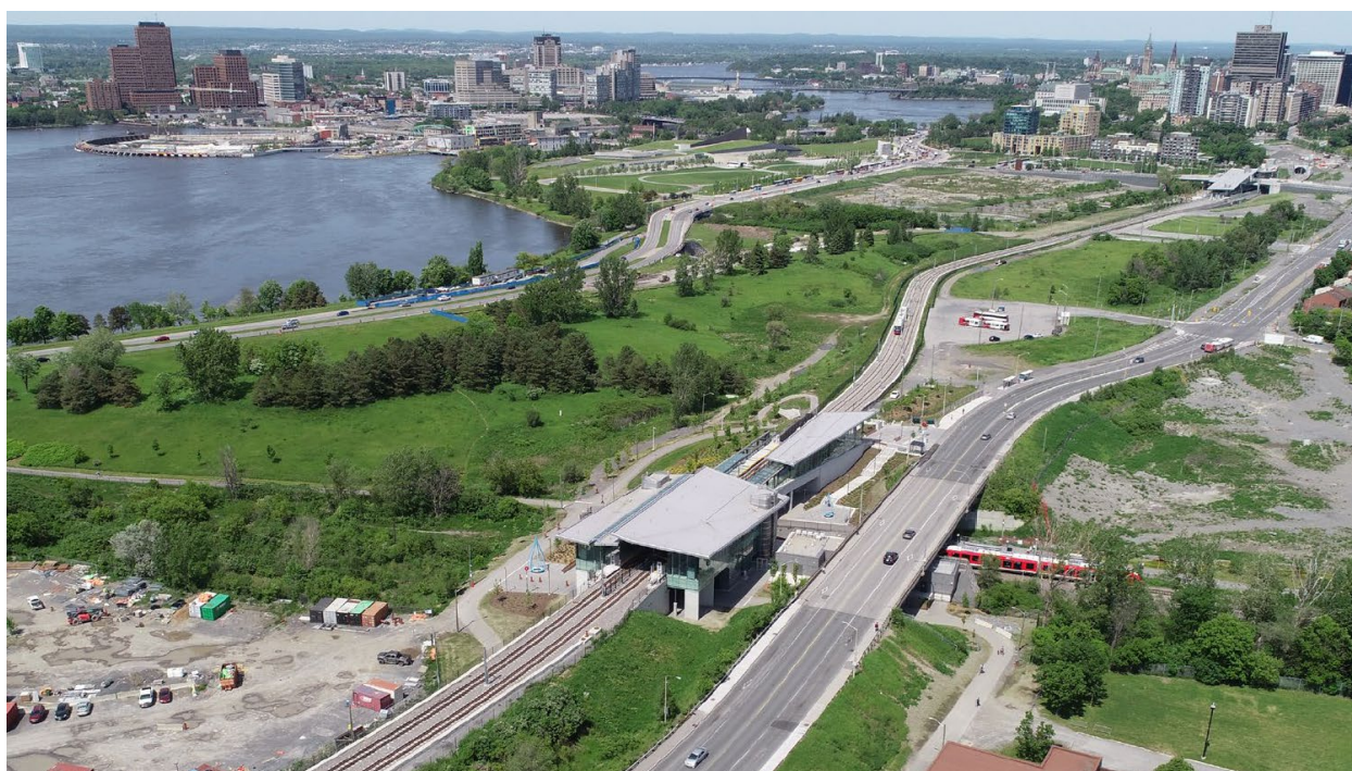
Figure 3-1: Aerial View of LeBreton Flats 3
