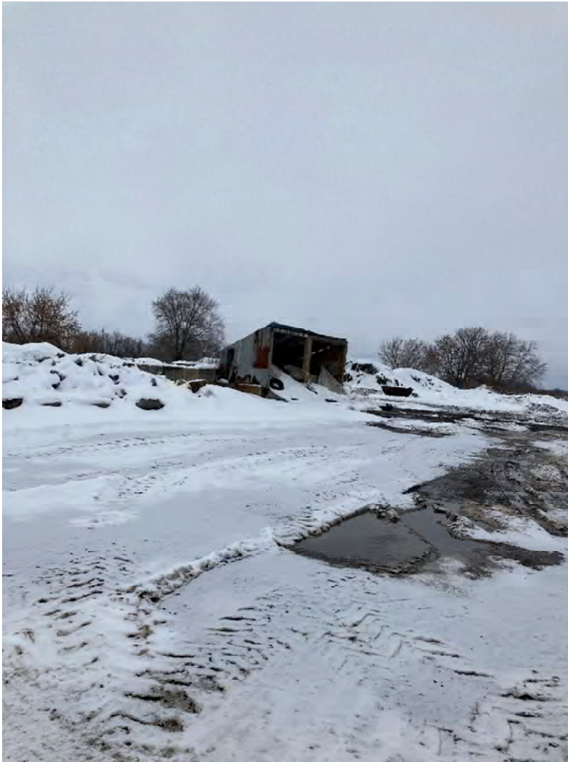
Photograph 7: Shed and fill material/debris found on the southeast corner of the Site.
