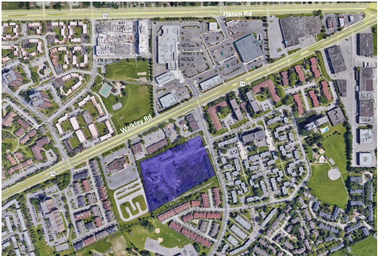
Figure 4 Aerial of proposed subdivision site (source: adapted from GoogleEarth Pro 2024)
