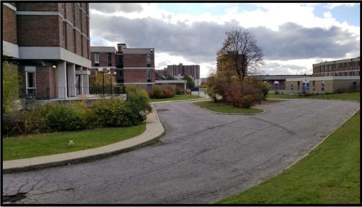
Photograph 3: View of the western portion of the Site, including Buildings K, J, and I (left to right, facing south).
