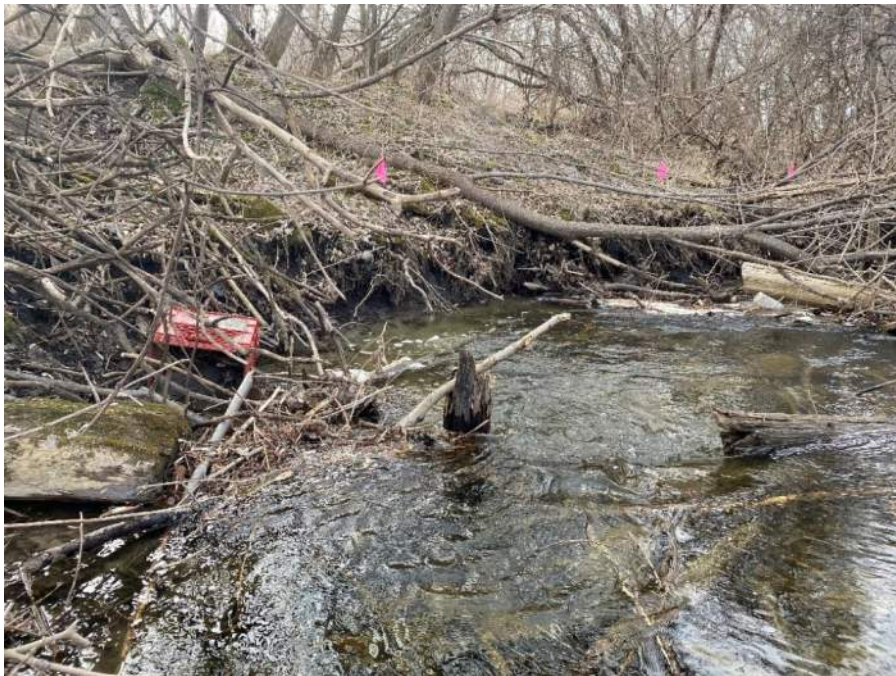
Toe erosion at the Poole Creek west of cross-section A
